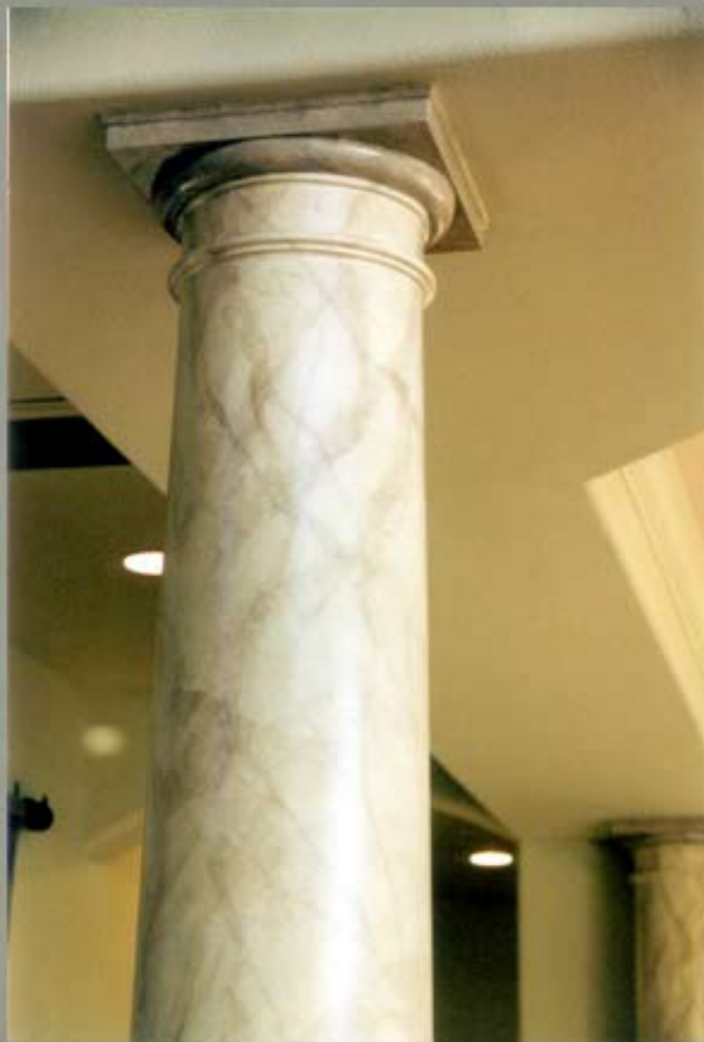
Marble columns at residence Santa Rosa, California.
